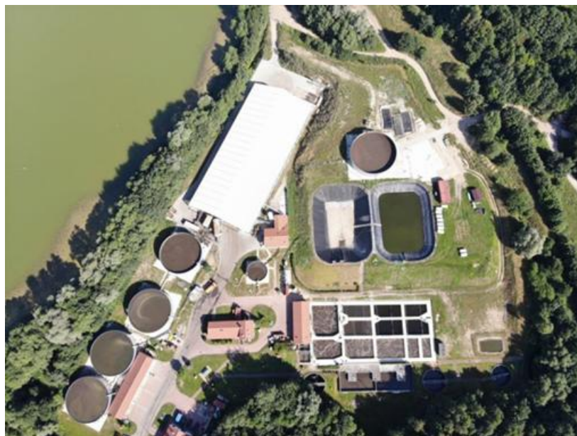
Figure b.28. Kartuzy WWTP aerial view during lake sediment treatment (Source: Kartuzy WWTP)
