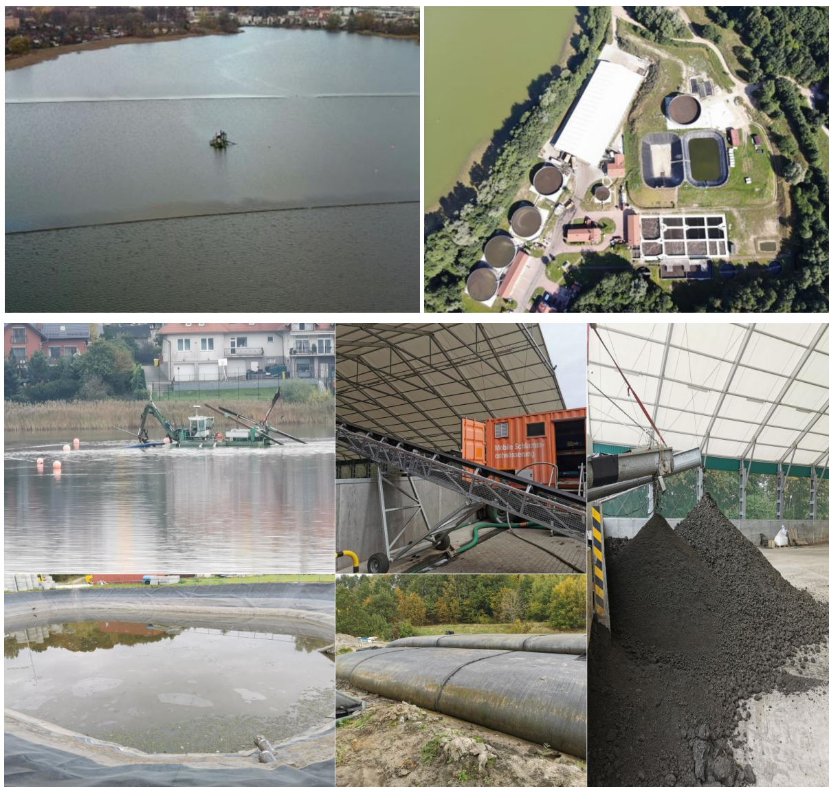
Figure 11 – Dredging at FutureLakes’ Kartuzy Demo Site and treatment of sediment at the Kartuzy Wastewater Treatment Plant. The sediment from Karczemne Lake was withdrawn by a dredger and transported directly to Kartuzy WWTP via pressure pipeline (length 4.5 km) in order to avoid leaks from the sediment storage on the shore of Karczemne Lake. Working sector in the lake was separated from the rest of the lake by geomembrane curtains. Kartuzy WWTP constructed full technological line for lake sediment treatment (several sedimentation tanks, screen grit chamber, centrifugation station and storage shed for final product of lake sediment treatment. © Kartuzy WWTP and Mike Lüring
