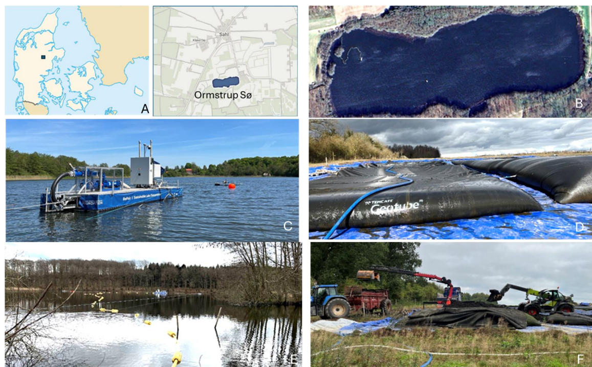
Figure 12 – Dredging at FutureLakes' Innovation Site Lake Ormstrup, Denmark and reuse of sediment on agricultural areas. A: location of Lake Ormstrup, B: satellite image of Lake Ormstrup where the dredger can be seen in upper left corner of the lake, C: the dredger, D: geotubes where the sediment is left for about ½ year for dewatering, E: pipe for sediment from dredger to land, F: removal and reuse of dried sediment from geotubes. © Martin Søndergaard
