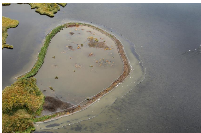
Figure 10 – Artificial reed beds and a central lagoon after construction at Hickling Broad, UK. Dredged sediment was diverted into geotextile tubes that were used in the construction of the artificial reed beds. © Mike Page
